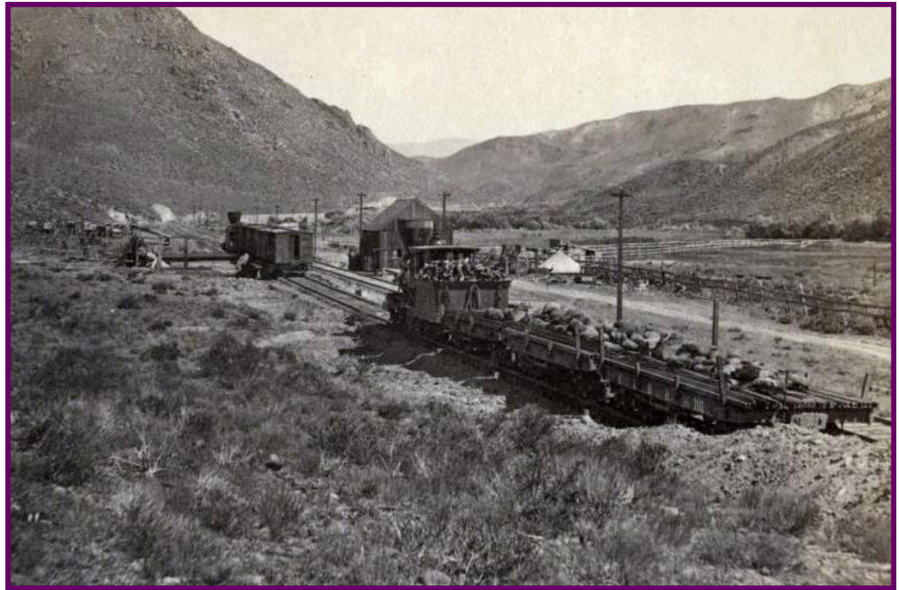
The Central Pacific entering the lower canyon of the Truckee River circa 1868, east of present day Sparks.. Alfred Hart photo.
