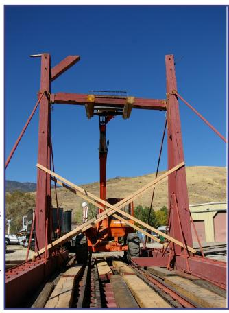
Shop staff remove the top sill of the A-frame after it became damaged in October 2014. (NSRM photo)
